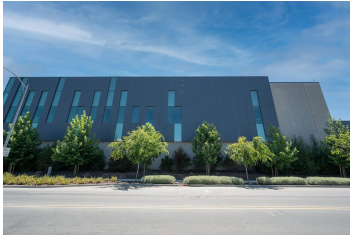
Equinix SV11 • San Jose Original Equinix project photograph
